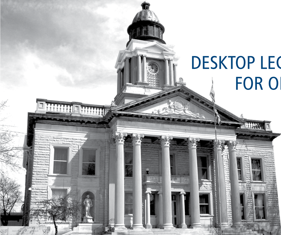
Crawford County Courthouse, Bucyrus, Ohio
