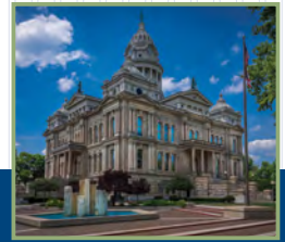
Miami County Courthouse, Troy, Ohio, Photo by David L. Dingwell
